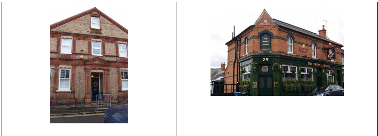
14 Alexandra Road/ 1 Albany Road corner terraced dwelling with highly decorative terracotta classical detailing - Prince Arthur pub displaying green glazed tiles and faience
