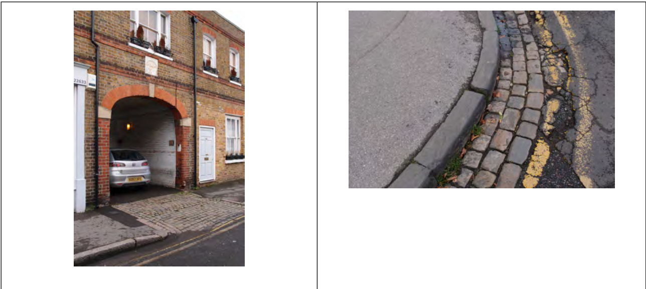
Stone sett entrance threshold on Grove Road and stone kerbs and stone sett gully
