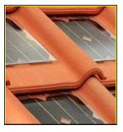
Already the appearance of photo-voltaic cells can be softened by embedding into clay tiles. It is to be hoped that technological development will further advance the provision of energy saving installations that conserve the appearance of historic tiled roofs.
