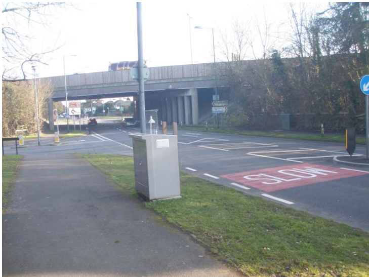
Figure 2.3 TRL monitoring station in Windsor Road
